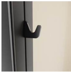
COAT HOOK At a height of 1200 mm / 47.24 in to ensure easy access for wheelchair users, promoting autonomy.
